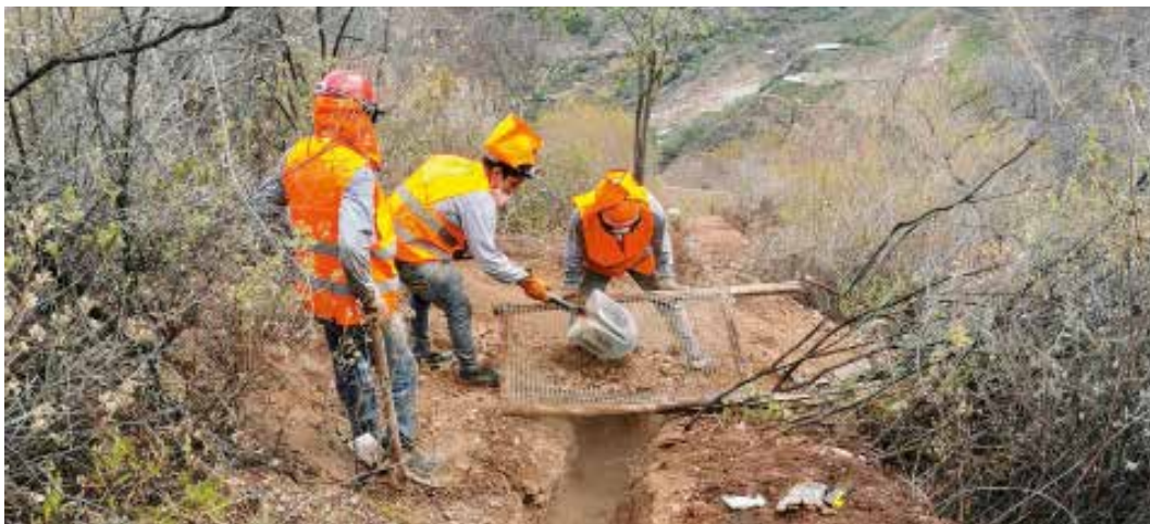
Covering the pipeline
