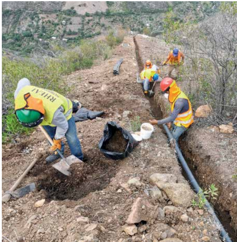
PVC pipeline installation
