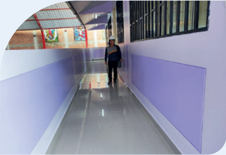
Classroom construction in Pueblo Nuevo community school, Pataz district.
