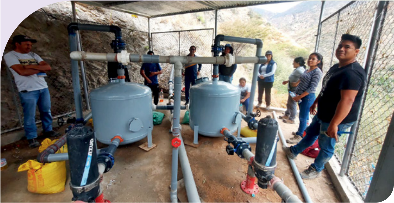
Improvement of the drinking water system in Vijus community, Pataz district.
